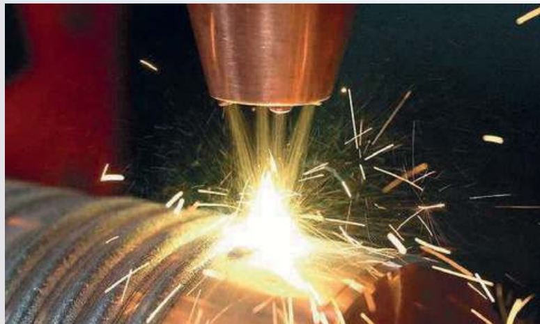
Restoration of shafts
